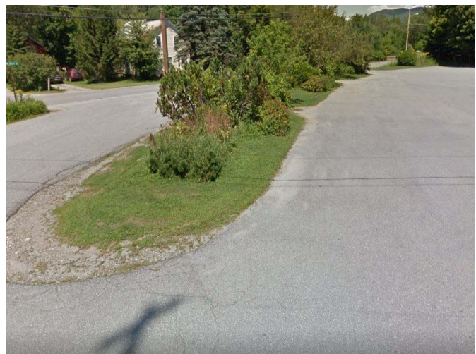
Figure 14. St. Thomas Church Parking Lot site. It is proposed that the existing swale be expanded and retrofitted as a bioretention to provide greater infiltration.
