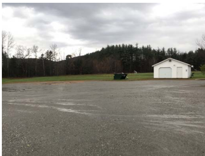
Figure 10. Subsurface infiltration chambers are proposed under the parking lot of the Underhill Central School.
