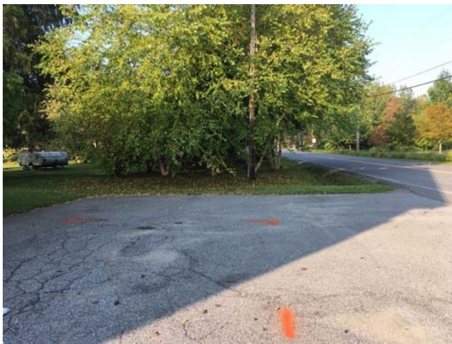
Figure 12. The Town Clerk's Office and Parking Lot site is the proposed location for a bioretention.
